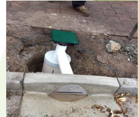
Kerb Inlet + Porous Well
